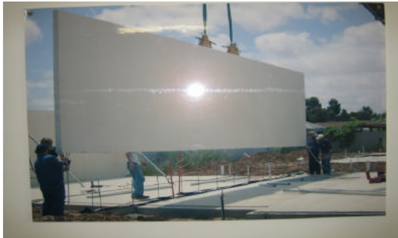
Fig.1 : Worlds' largest load bearing lightweight panel being used in Australia
