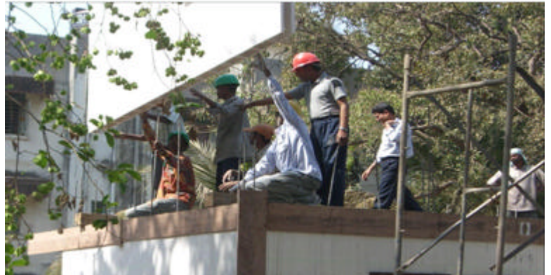
Fig 8 : Erection of upper floor panel
