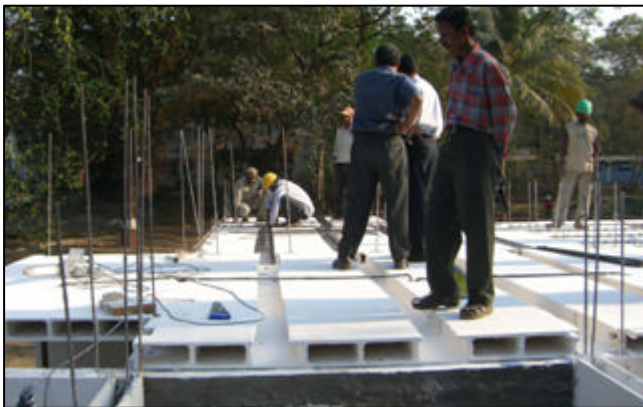
projection. Fig 6 : Cutting of top flange
